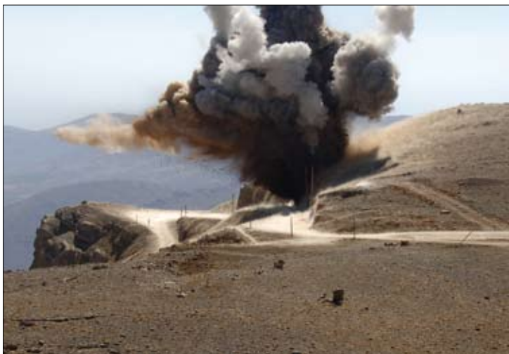
Blasting of the hanging Rock "Felsenkopf" in the AOR of the 1st Coy
